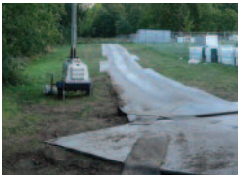
Use temporary tracking to prevent rutting and compaction in car parking areas.
